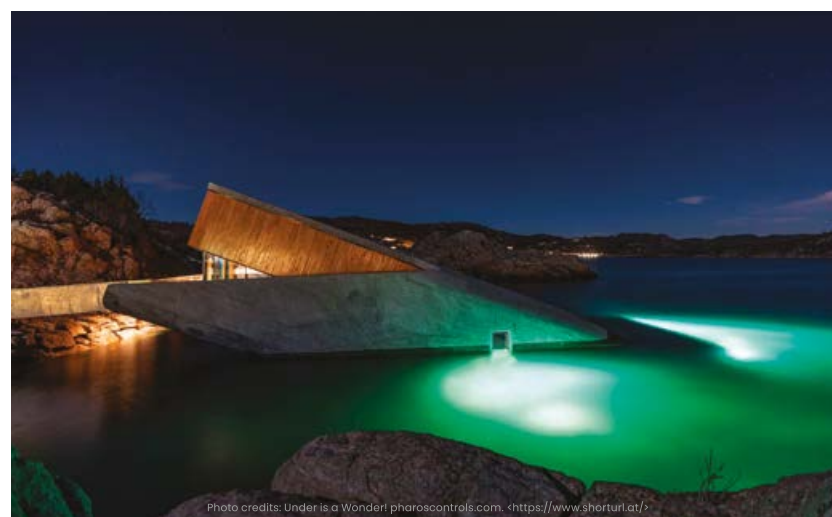
Photo credits: Under is a Wonder! pharoccontrols.com, <https://www.shorturl.at/>
